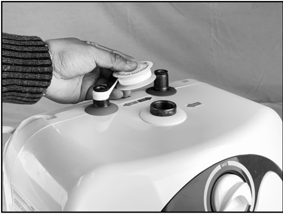
STEP 15: Cover both threads of the water heater.
