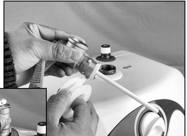
STEP 16: Cover with teflon as well the pressure valve thread. Use a pipe pliers to install it as shown in the image.
