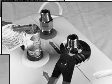
STEP 17: Install 1/2" couplers on both threads of the water heater. Use pipe pliers to fully tighten. Cover the coupler threads with teflon tape as shown.
